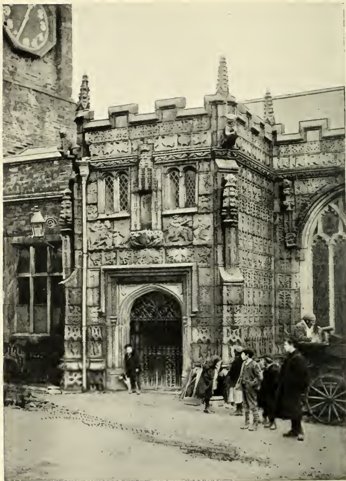
LAUNCESTON CHURCH PORCH
